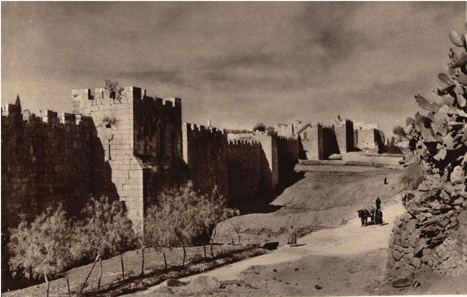
Figure 8. Northern wall of Jerusalem, Photograph by Ludwig Preiss. 1926. Courtesy of Piki Wiki Israel.
